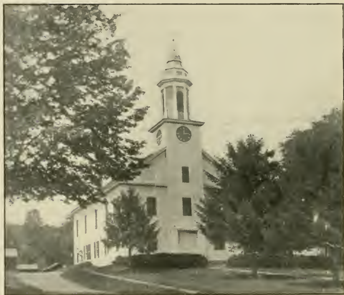
CONGREGATIONAL CHURCH SOUTHAMPTON, MASS. ERECTED 1788
